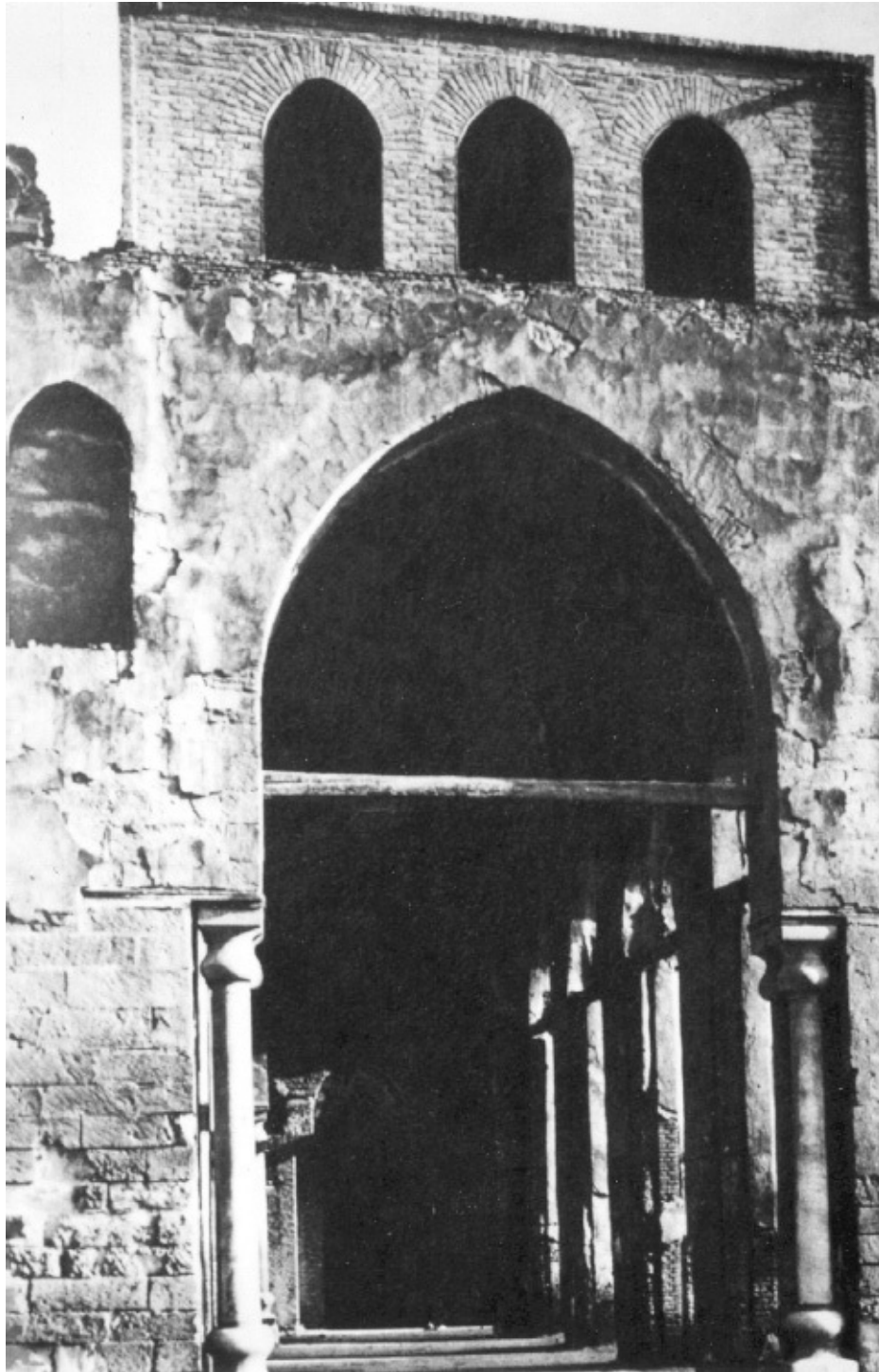
Figure A2.E. The Cairo Mosque of al-Hakim ca. 690 CE
